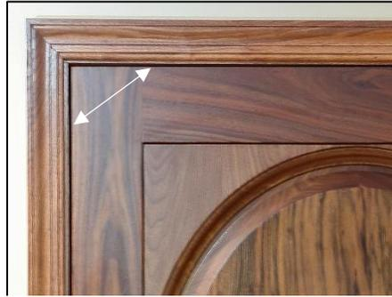
Figure 3 – Checking Door Spacing
